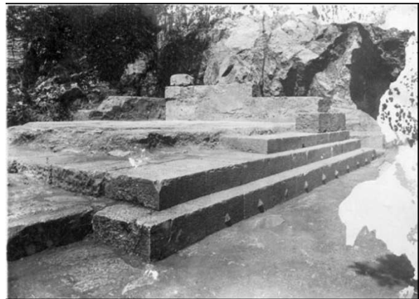
Fig. 8 : Temple above the theater (with lifting bosses)
