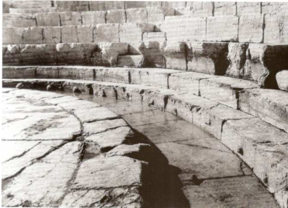
Fig. 9. Theater, lowest course with lifting bosses.
